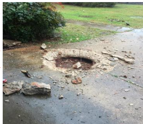
A lightning strike caused extensive damage to this driveway in Magee, MS. Photo by Chris Curlee
