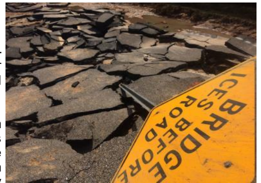
The aftermath of river flooding along Black Creek at Hwy 589 in Lamar County, from March 8-13, 2016. Photo by Lamar EOC
