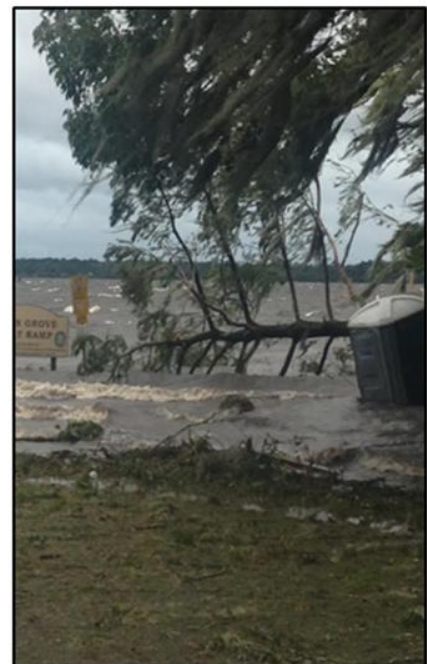
Eglin Grove Boat Ramp inundation
