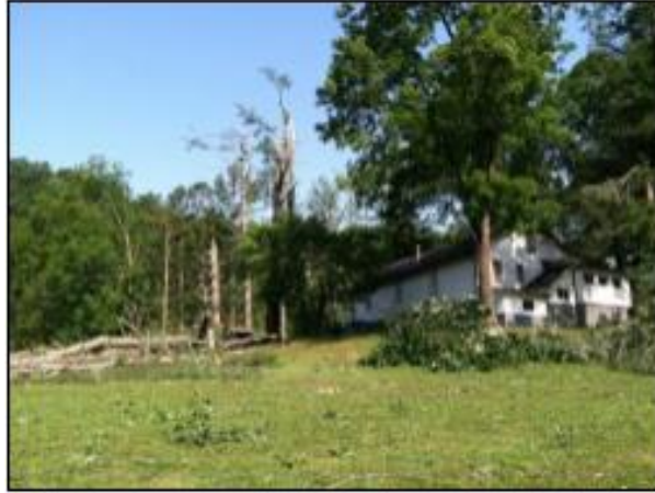
Figure 4: Damage from wind at Camp Nathaniel on July 5th.
