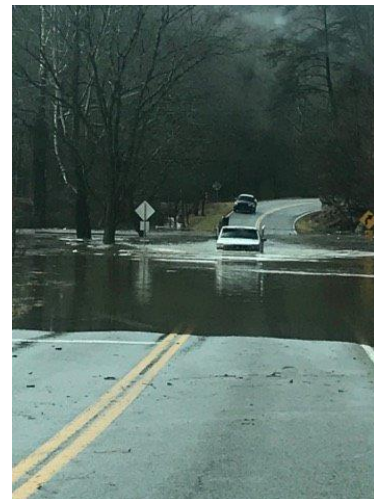
KY Highway 7 in Letcher County. Picture courtesy of Sheena
