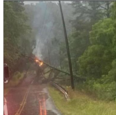
Tree on Power Line in Elna Courtesy of Big Sandy RECC
