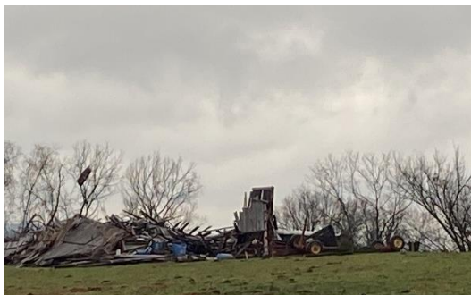
Destroyed barn in Estill County Courtesy of National Weather Service, Jackson
