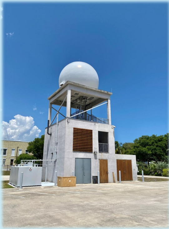
RRS antenna dome in the backyard of the Florida Keys NWS office.
