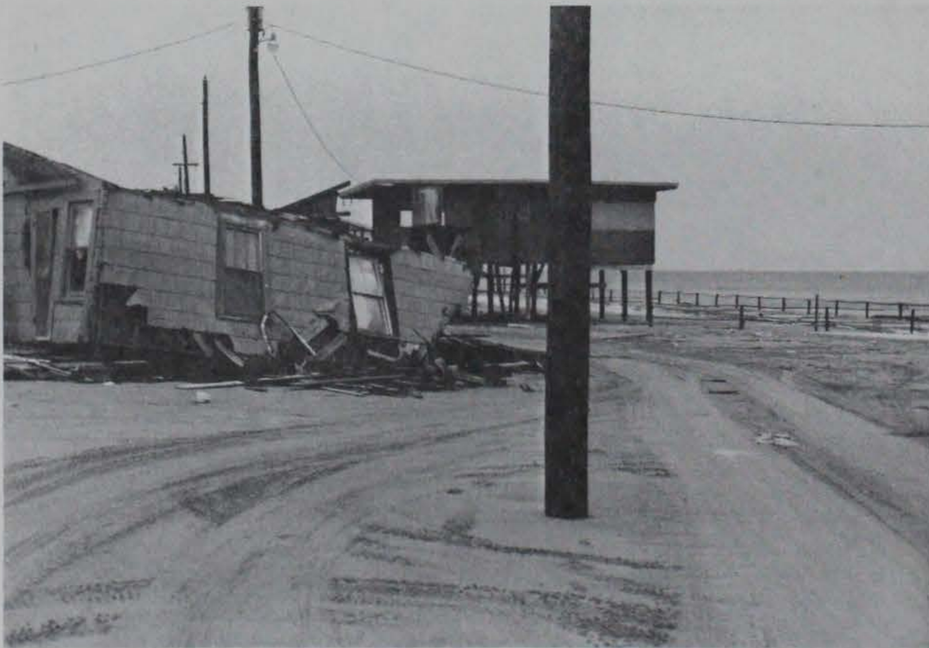
Figure 7. Damage from Tropical Storm Chris in Holly Beach, Louisiana
