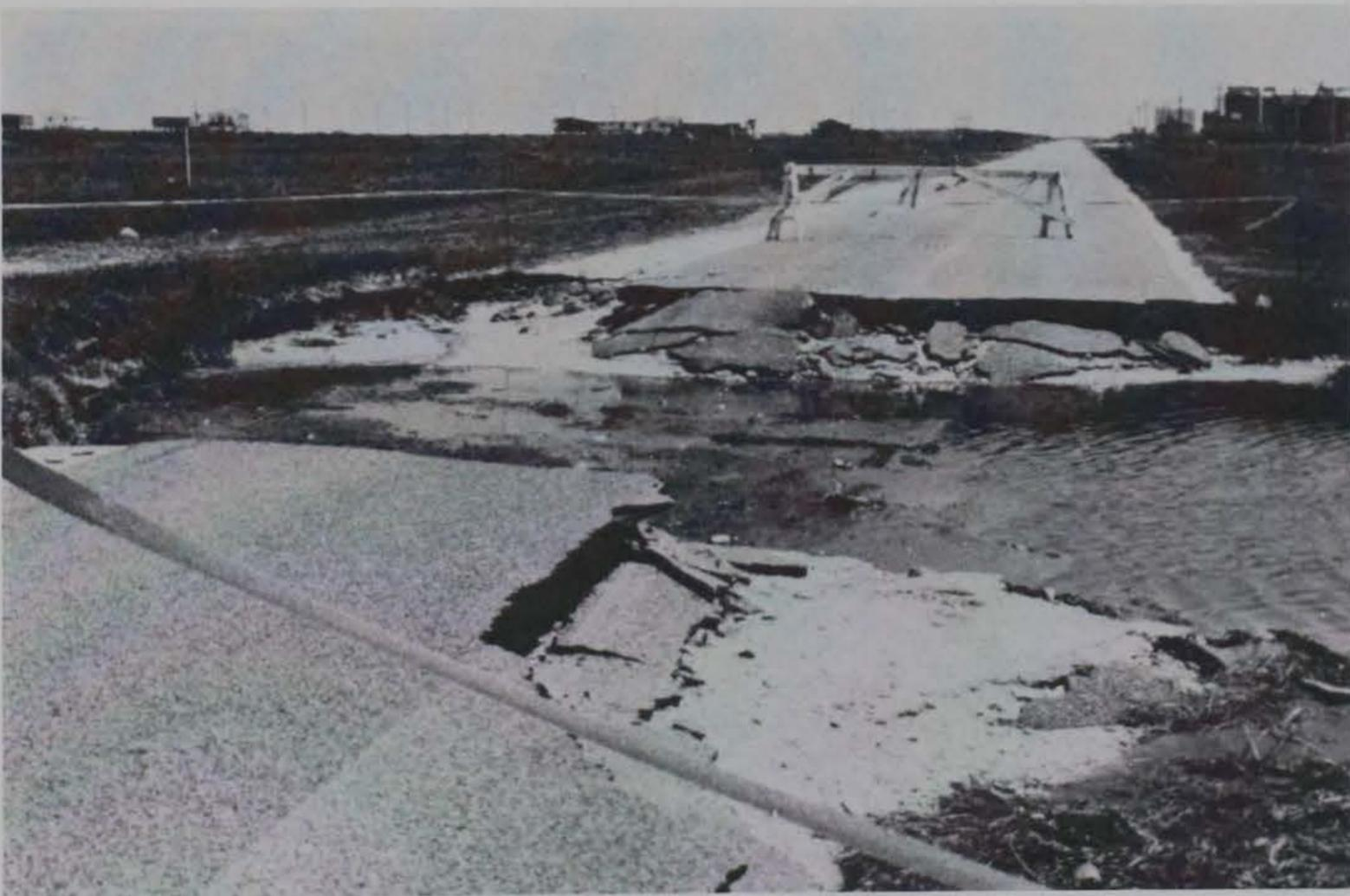
Photo 4. Highway damage near eastern end of Follets Island
