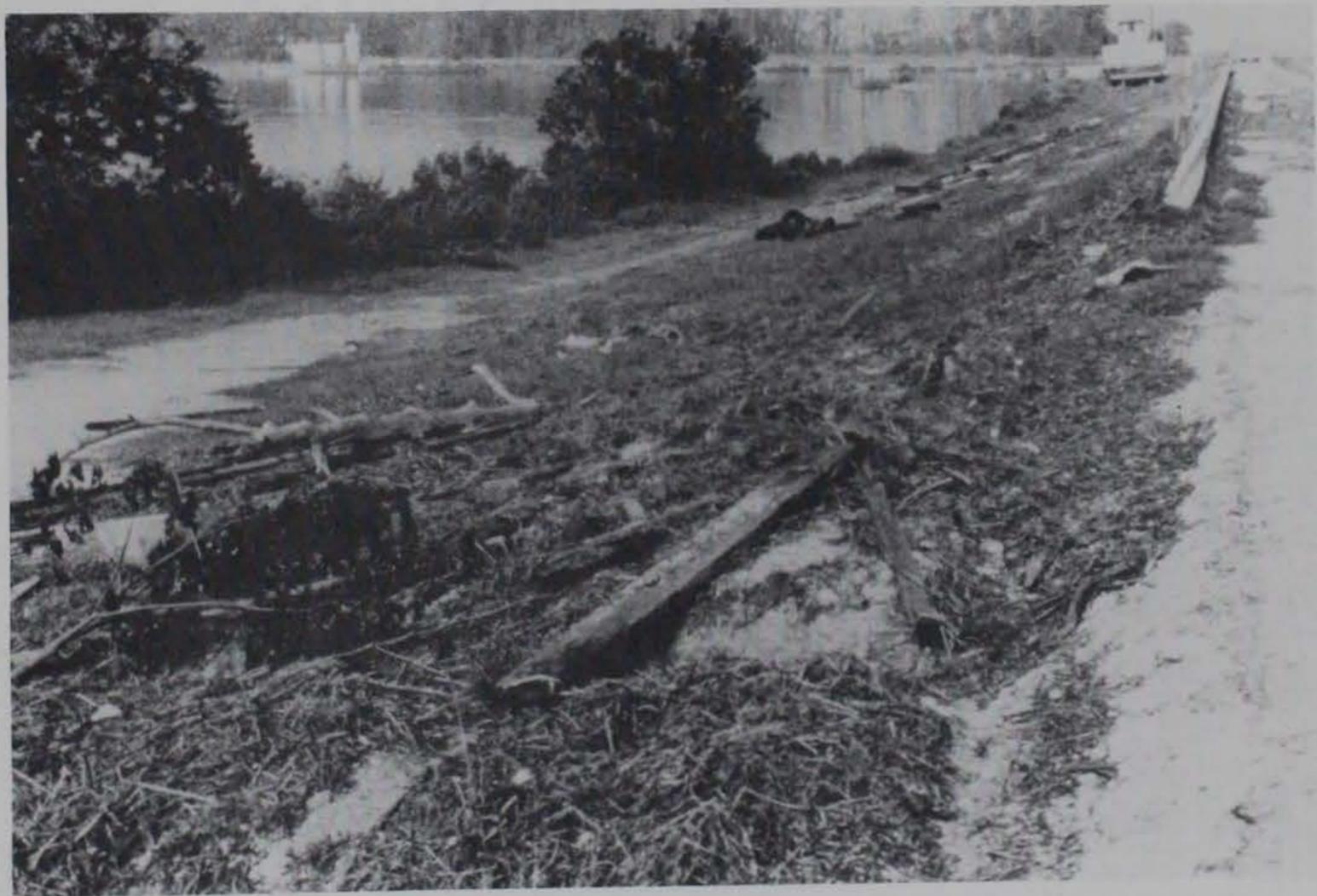
Photo 12. Debris line and stranded tug on Highway 146 embankment, Baytown, Texas
