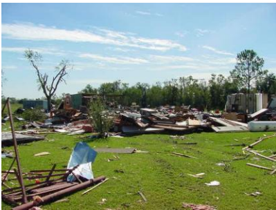
Tornado damage in China, TX
