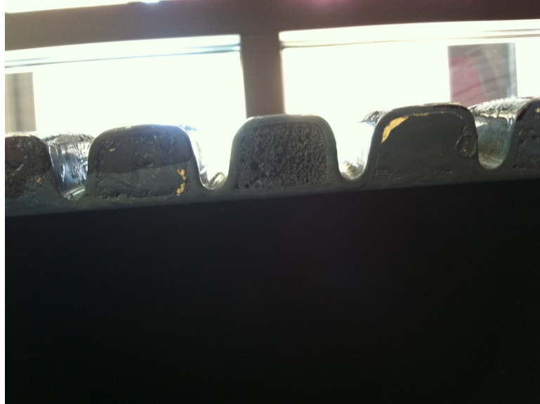
Above: Sealant foam filling in the holes in the corrugation.
