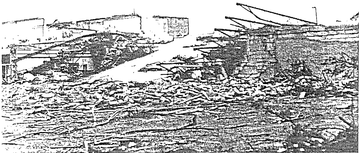
FIGURE 53. XENIA HIGH SCHOOL, CAFETERIA. Roof collapsed when loadbearing masonry walls failed.
