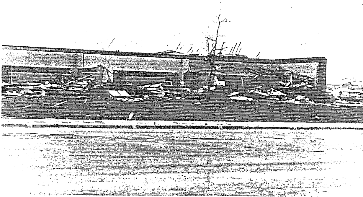
FIGURE 42. SIMON KENTON ELEMENTARY SCHOOL, CLASSROOMS. Exterior walls had collapsed and the roof was entirely uplifted.
