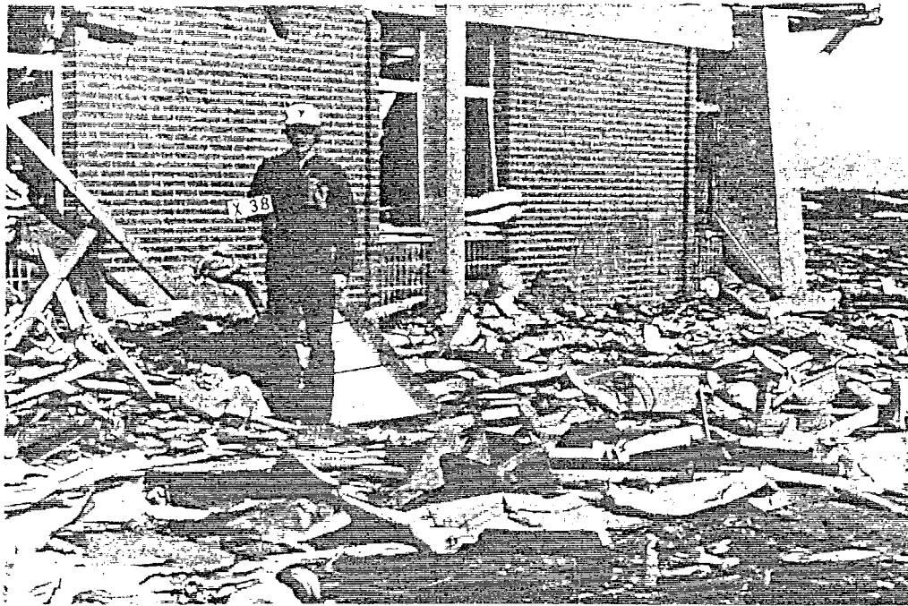
FIGURE 65. DEBRIS. Pieces of timber, roofing material, and other small items deposited at the corner of Arrowood Elementary School. This type of accumulation of debris was typical along the path of the tornado through residential areas.
