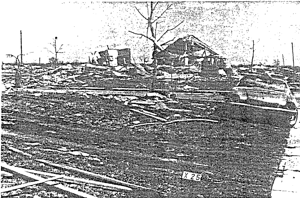
FIGURE 64. RESIDENCE IN SOUTHWEST XENIA. The residences were damaged beyond repair, although there remained some walls standing in most of them.
