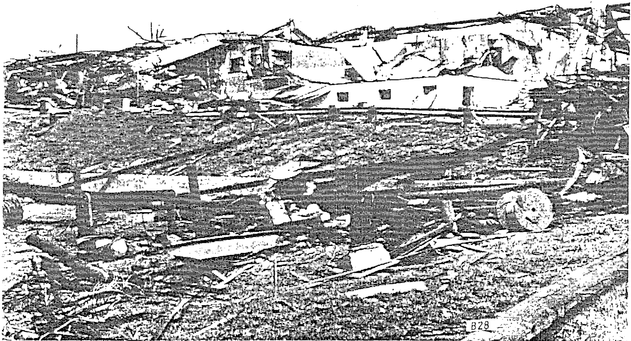
FIGURE 78. REC HEADQUARTERS. The utility poles were stored on the rack in the foreground. Although in an ideal position to become airborne, the poles did not move beyond what is shown in the photo.
