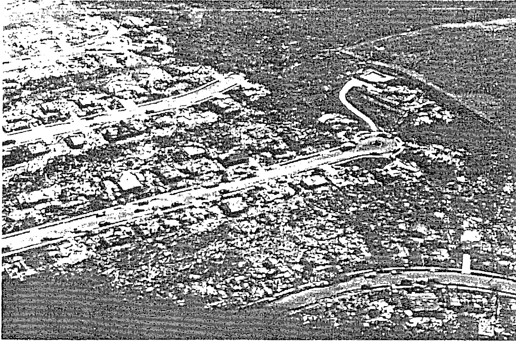
FIGURE 63. RESIDENCES IN NORTHEAST XENIA. The path of the tornado is from bottom right corner to the top left corner. Most of the homes were damaged beyond repair.
