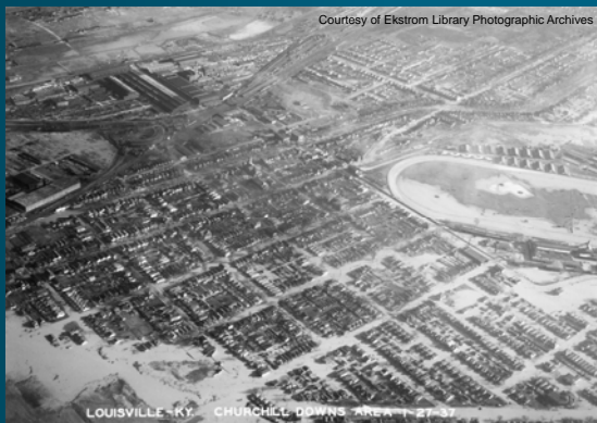
Widespread flooding at and around Churchill Downs.
