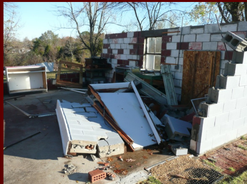
A Tornado Warning was in place for nearly ten minutes before the tornado that did this damage struck near Mount Washington, Kentucky on October 26.
