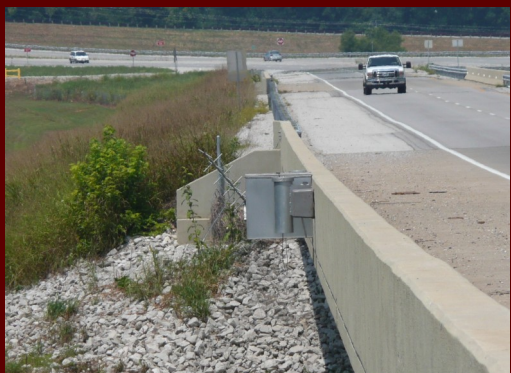
River gauge equipment on the side of the US 231 bridge over Drakes Creek near Alvaton, Kentucky.
