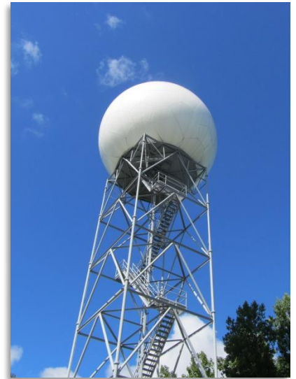
NWS radar tower at Fort Knox. The antenna spins inside the white ball at the top.
