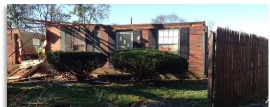
EF-1 damage to a home found during a storm survey in Paris, KY after the October 7 tornado.
