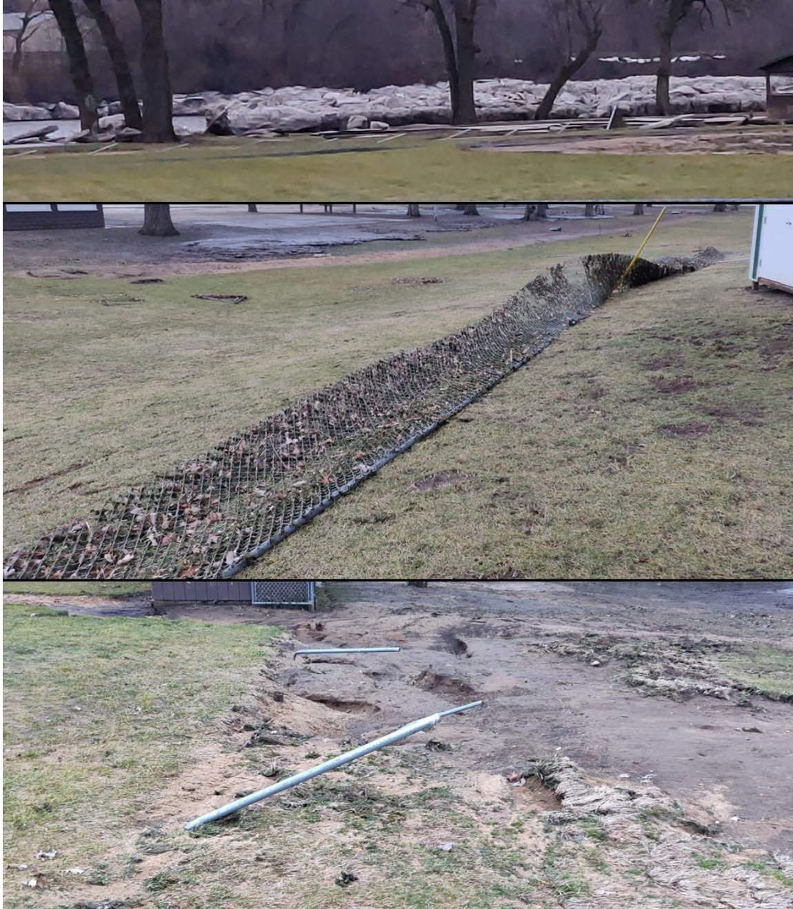
Figure 18. Chain link fencing damaged at the north (downstream) end of Island Park in Wilmington due to flooding and ice flows. Photographed on January 30.
