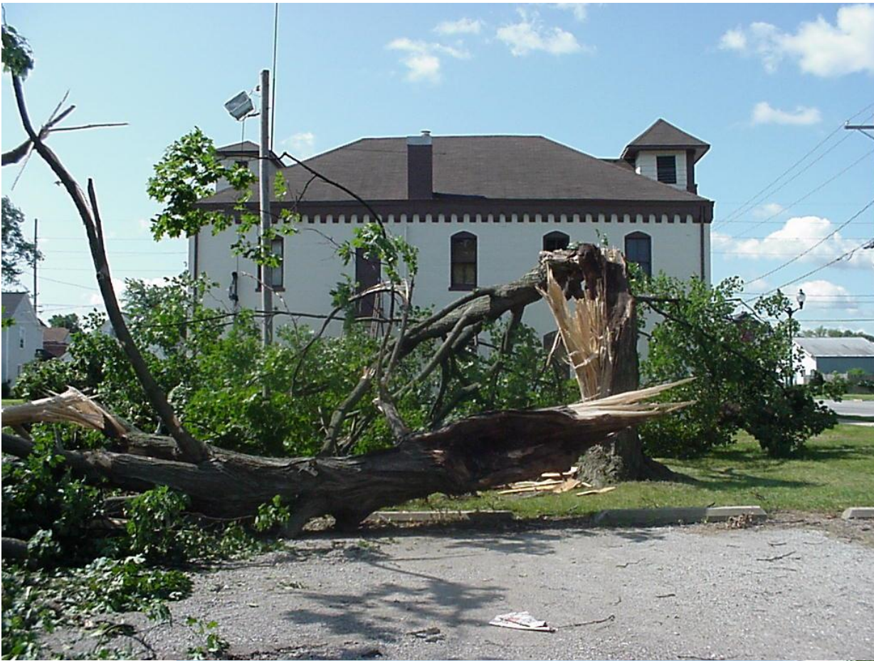
Tree damage near the west side of the O'Fallon, Illinois Police Department complex. Viewing south.
