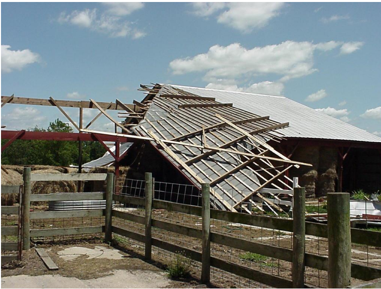
Damage to a machine shed on a farmstead 1 mile west of Lebanon, Illinois. Viewing north.
