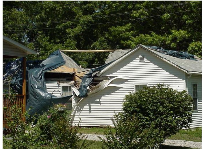
Damage to one of several homes due to fallen trees in the town of Trenton, Illinois. Many of the trees were originally 40 to 50 feet tall. Viewing northeast.
