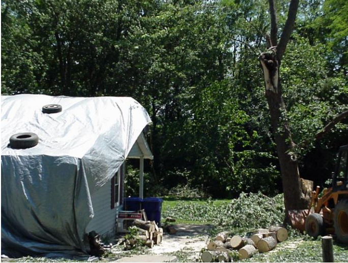
Damage to one of two homes over the southern part of the town of Summerfield, Illinois. The west side of the roof from this home is severely damaged. Viewing south. Several large trees were uprooted southwest from this location.
