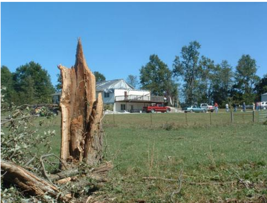
EF1 Tornado damage near the intersection of Highways CC and 15 in Monroe County.
