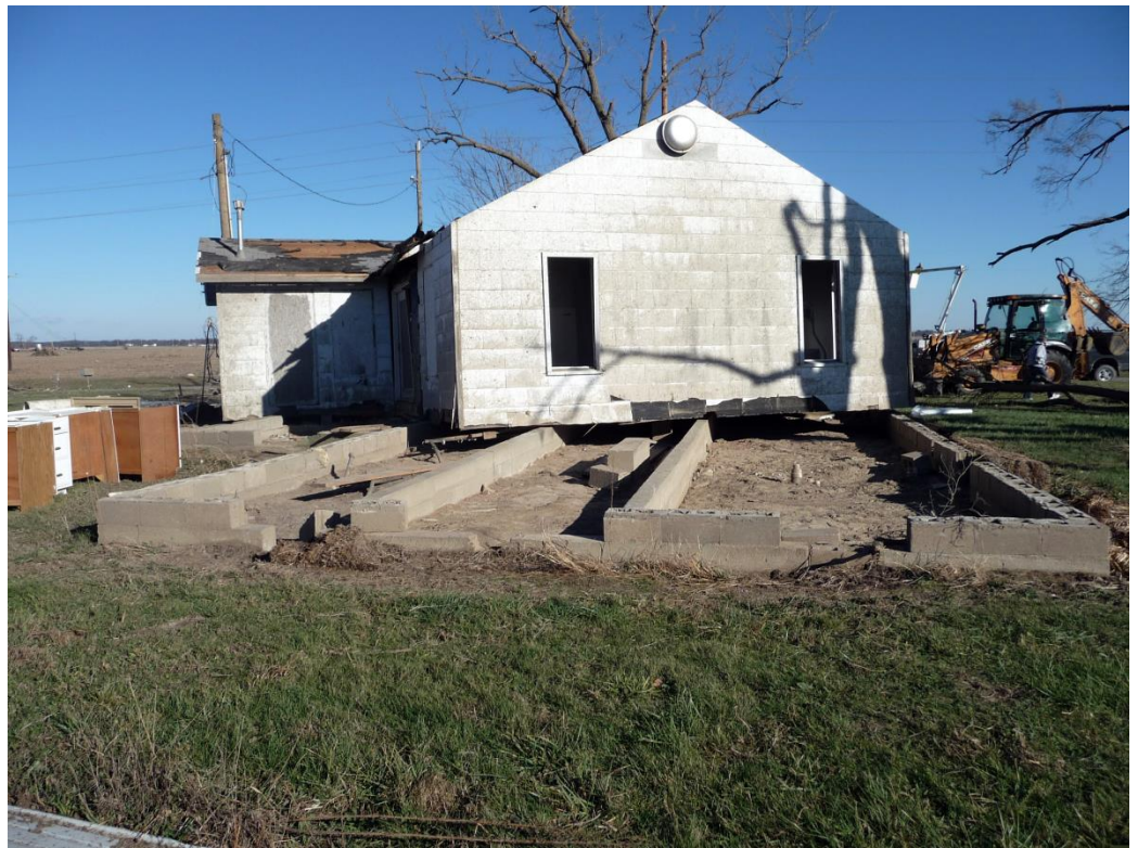
Tornado damage to a house west of St. Elmo, Illinois.
