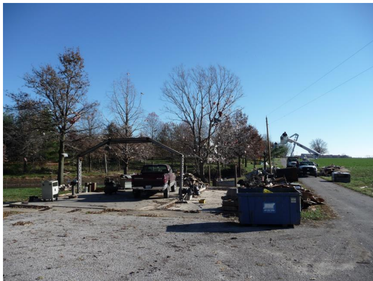
Tornado damage to a garage along Low Bridge Road east of Jamestown Road (north of Breese, Illinois)
