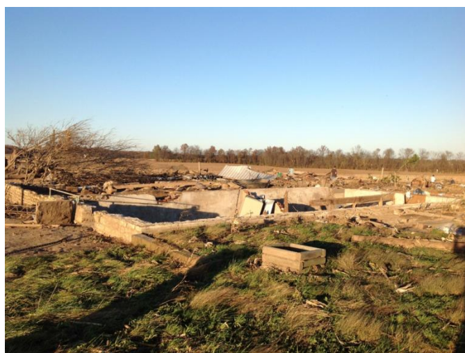
A farm house was completely swept clean from its foundation. This damage was rated EF4. Two fatalities occurred at this location.
