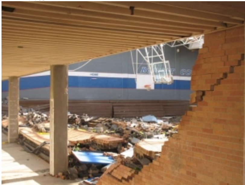
The Childress High School suffered a direct strike by an F2 tornado during the evening of the 9th. Several million dollars worth of damage was sustained at the school district's facilities. A 109 MPH wind gust was recorded as the tornado moved across the campus. The gymnasium (pictured above) was destroyed. Photo courtesy: National Weather Service - Lubbock, Texas.
