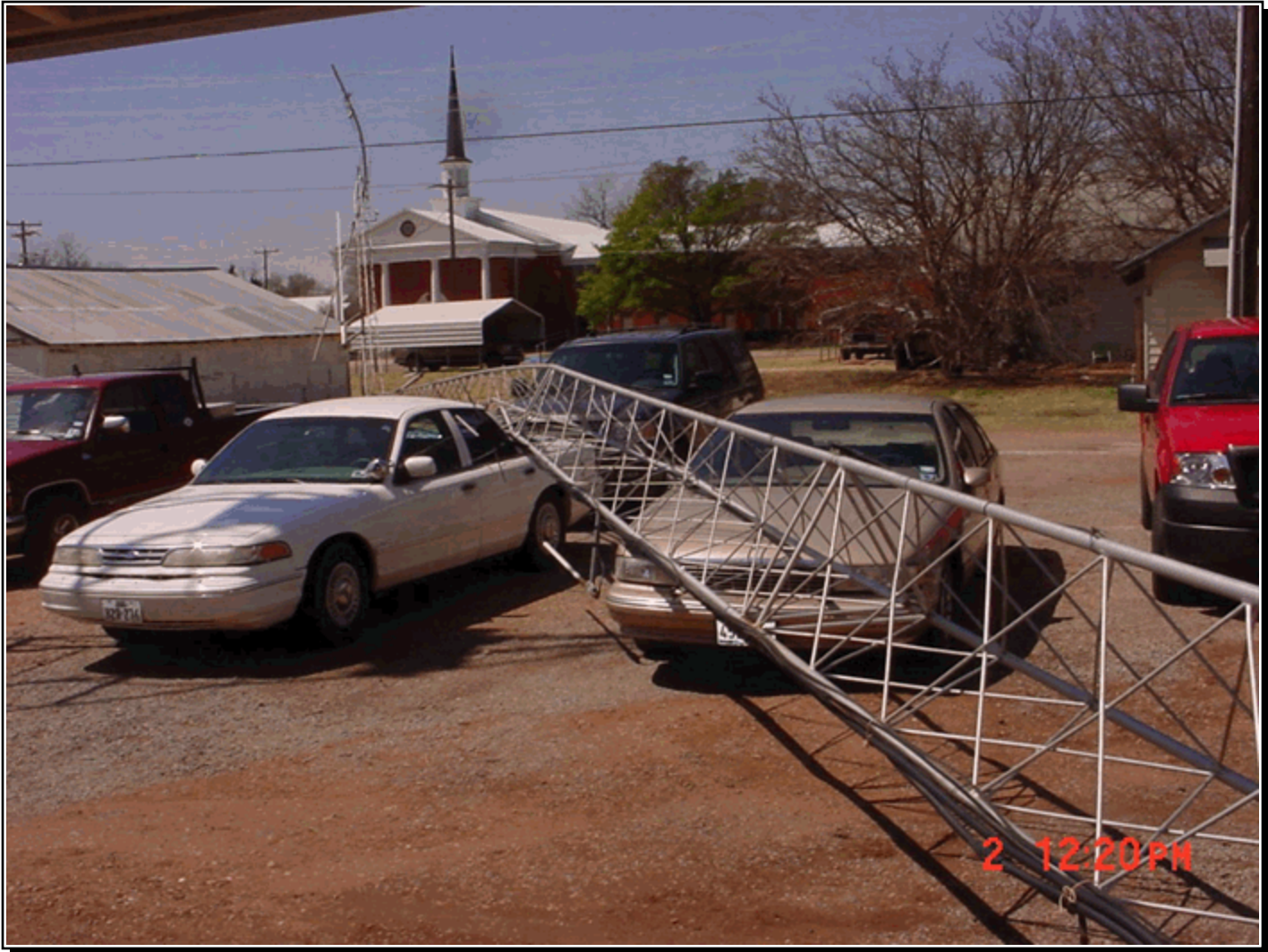
High winds downed a 100 foot radio communications tower in Paducah (Cottle County) during the morning hours of the 2nd. The tower fell onto and damaged cars in a parking lot. Photo courtesy: Randy Detwiler - Paducah Fire Department.
