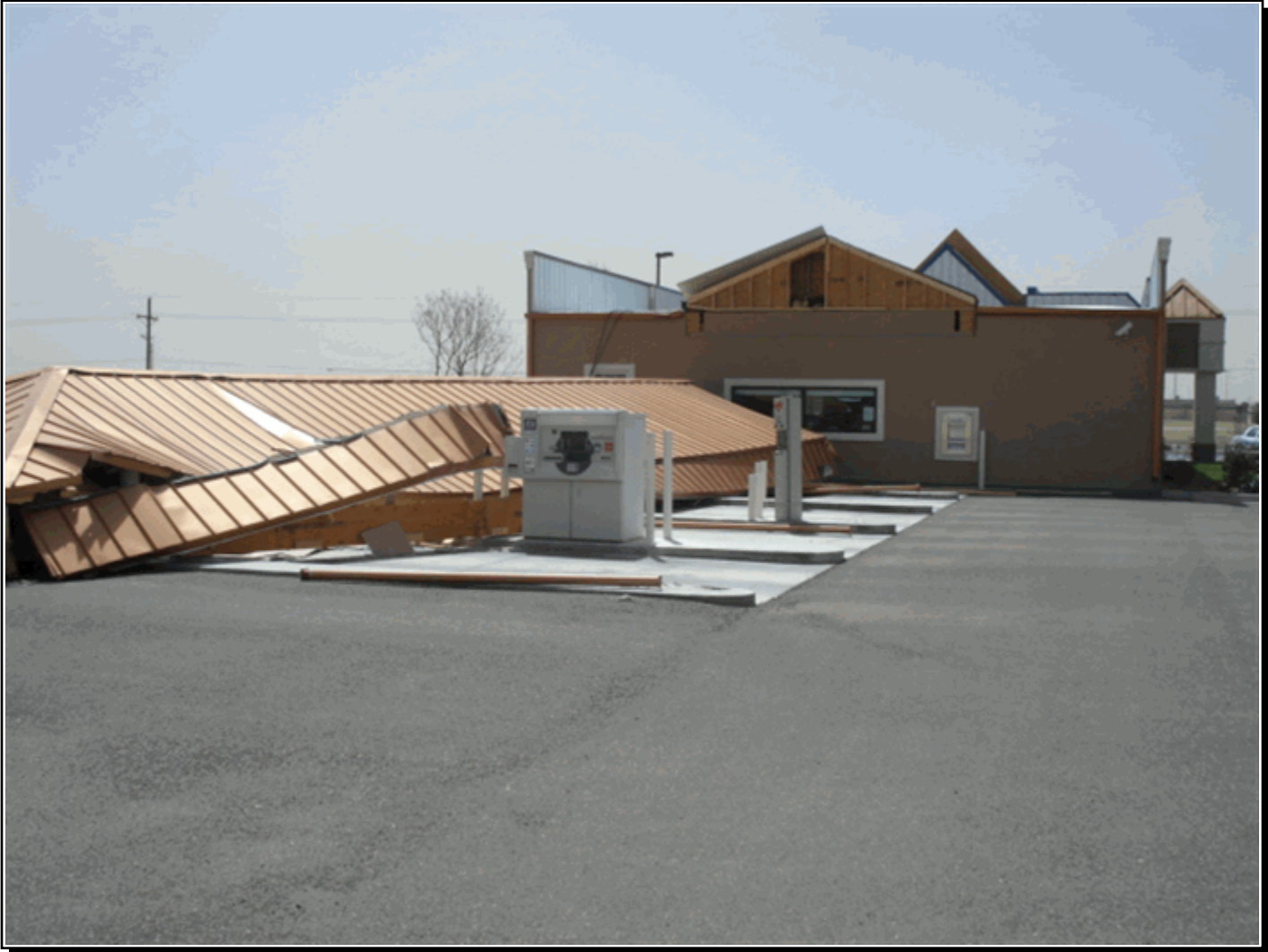
A bank teller awning was destroyed by high winds in Wolfforth (Lubbock County) shortly before noon CST on the 9th. Photo courtesy: Karen Michael - FrenshipToday.com
