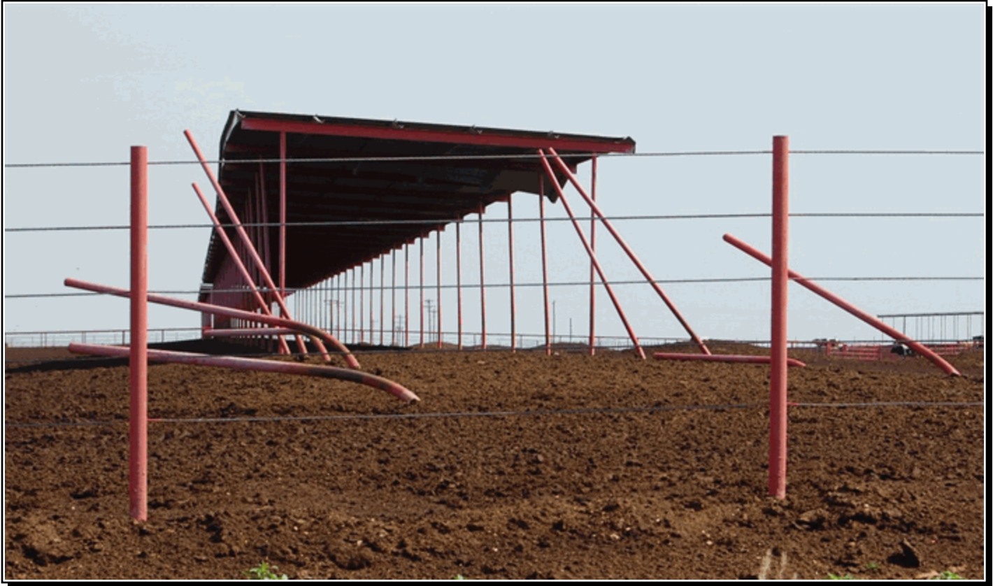
A portion of a large livestock shade about 2.5 miles southwest of Hart was blown away by winds estimated around 70 mph. Photo courtesy of NWS COOP Observer Neoma Williams.
