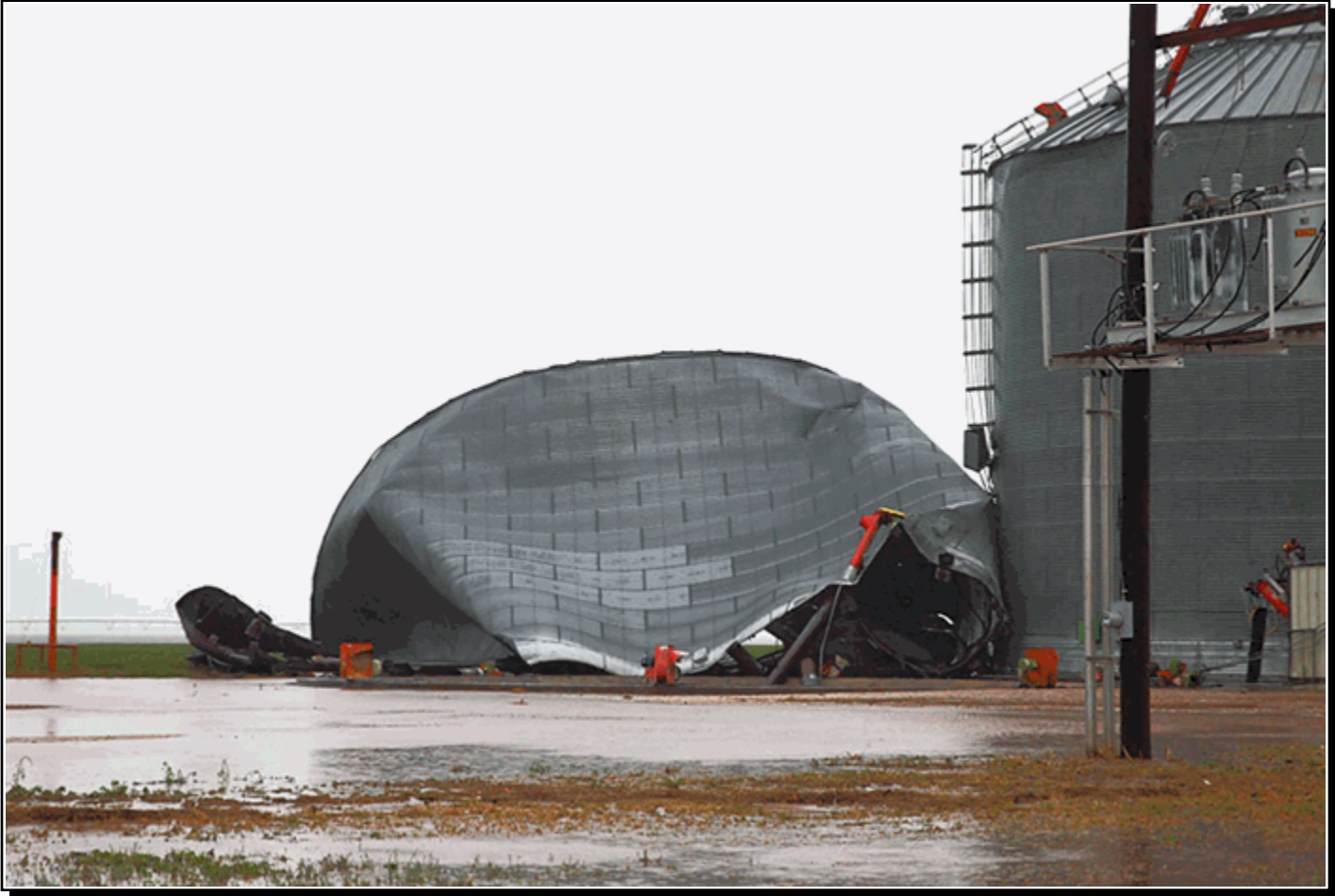
Downburst winds estimated around 90 mph severely damaged this large grain storage bin in Flagg. Photo courtesy of Matt Ziebell.
