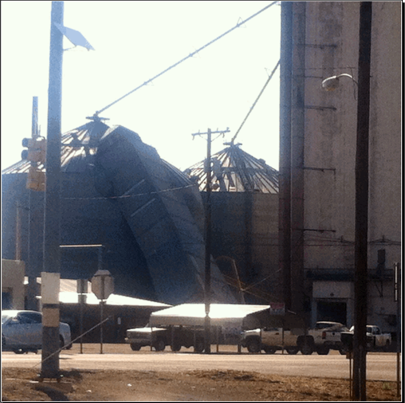
A grain dryer in Hart blown over against a grain tank by thunderstorm downburst winds. Photo courtesy of Brad Barnes with the Hart Fire Department.
