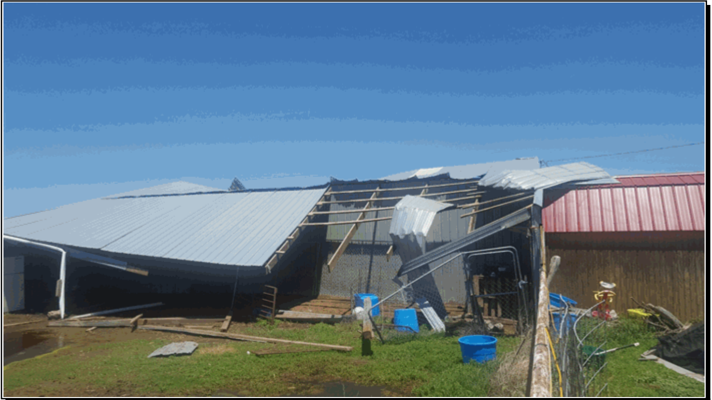
Photograph of a metal barn that was partially destroyed by rear flank downdraft winds. Photograph taken by the NWS storm survey.
