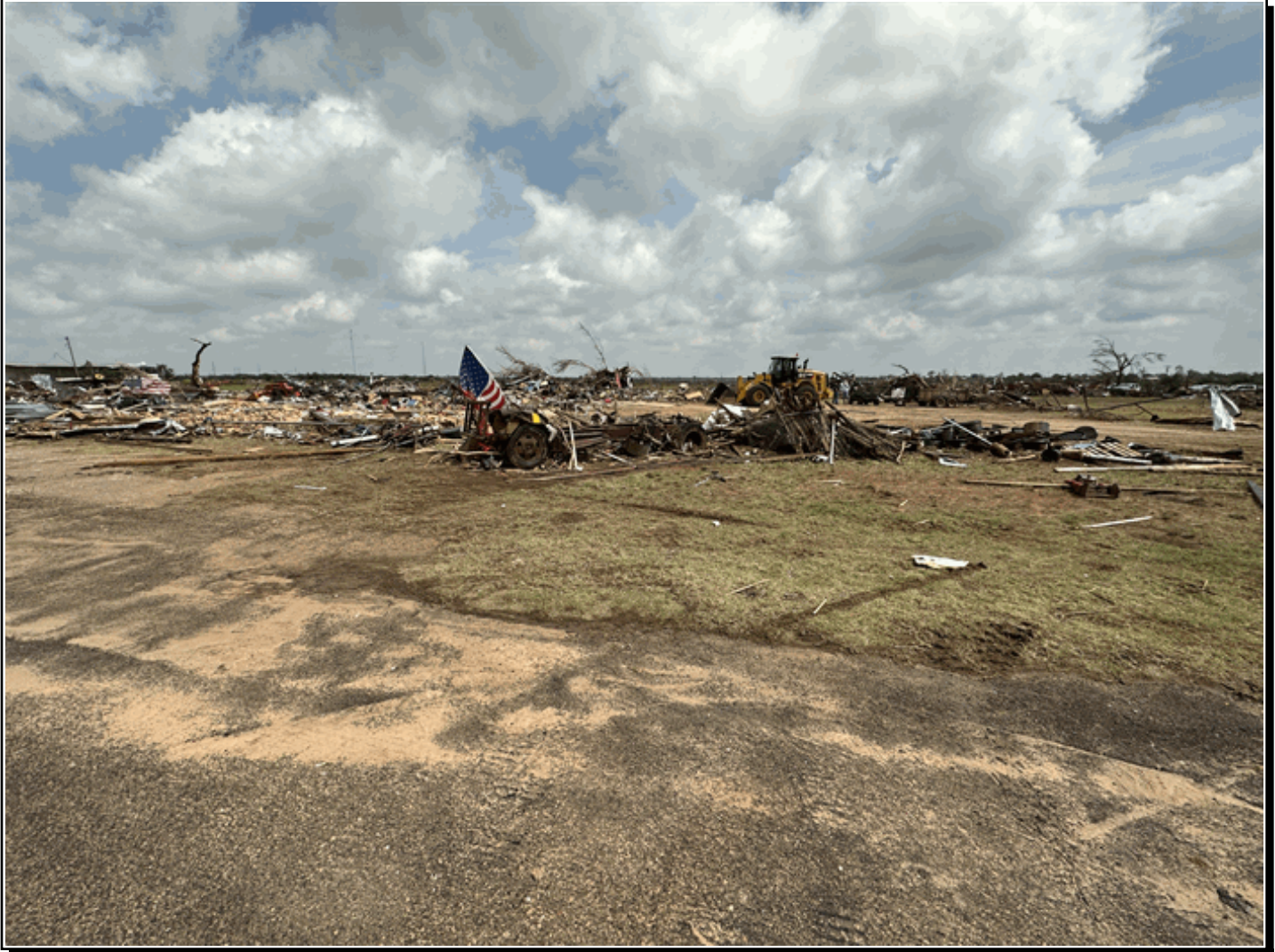
Widespread severe damage and ongoing cleanup on the west side of Matador the day after a tornado hit town. Photograph from the NWS storm survey team.
