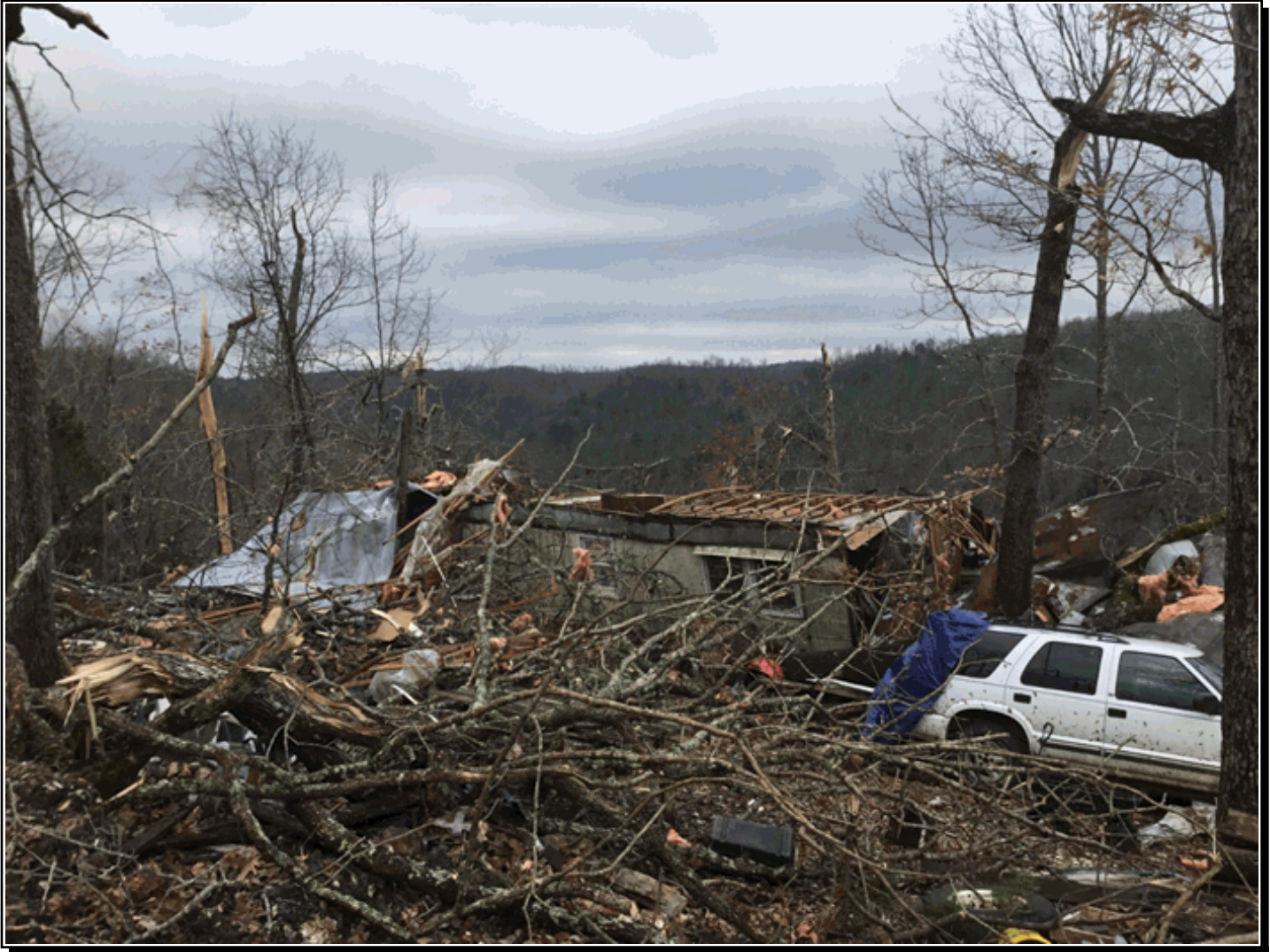
A mobile home was severely damaged from an EF1 tornado near the end of Crestwood Terrace Road east of State Hwy 14 in southern Marion County during the morning hours of February 7th. The sole injury from this tornado occurred at this residence. Photo courtesy of the National Weather Service Little Rock, AR.
