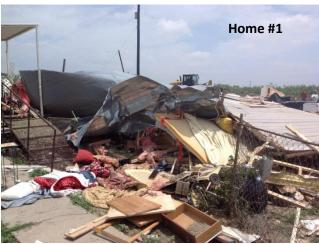
Tornado #7 developed around at 8:56 PM CDT, just over 1 ½ miles NNW of Garden City. This tornado produced a combination of EF1 and EF2 damage at two residences. A single-wide manufactured home at Home #1 was rolled and destroyed. This was indicative of damage produced by a tornado of EF2 intensity. As the tornado moved southwestward and impacted Home #2, a combination of EF1 and EF2 damage was noted. Tree damage was indicative of EF1, while the metal barn appears to
