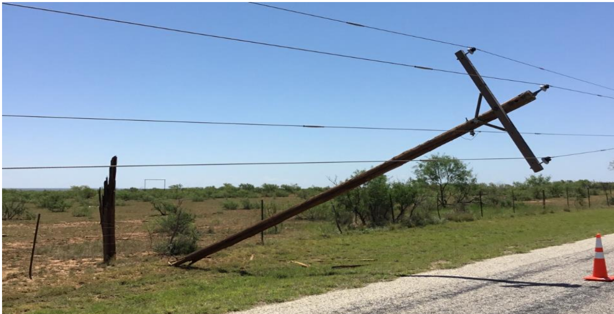
Figure 7: This pole was the furthest south on Willow Valley Road and was snapped near the base of the pole.
