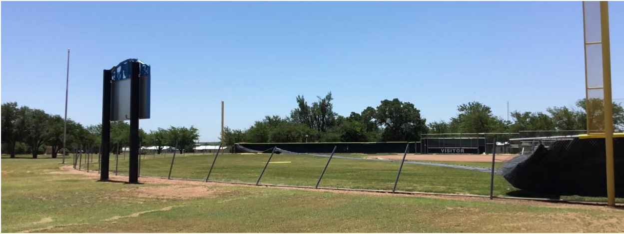
Figure 4: This is a photo of the softball field at Borden County School. The metal poles were all bent towards the southeast, and the fencing along the poles was ripped off.
