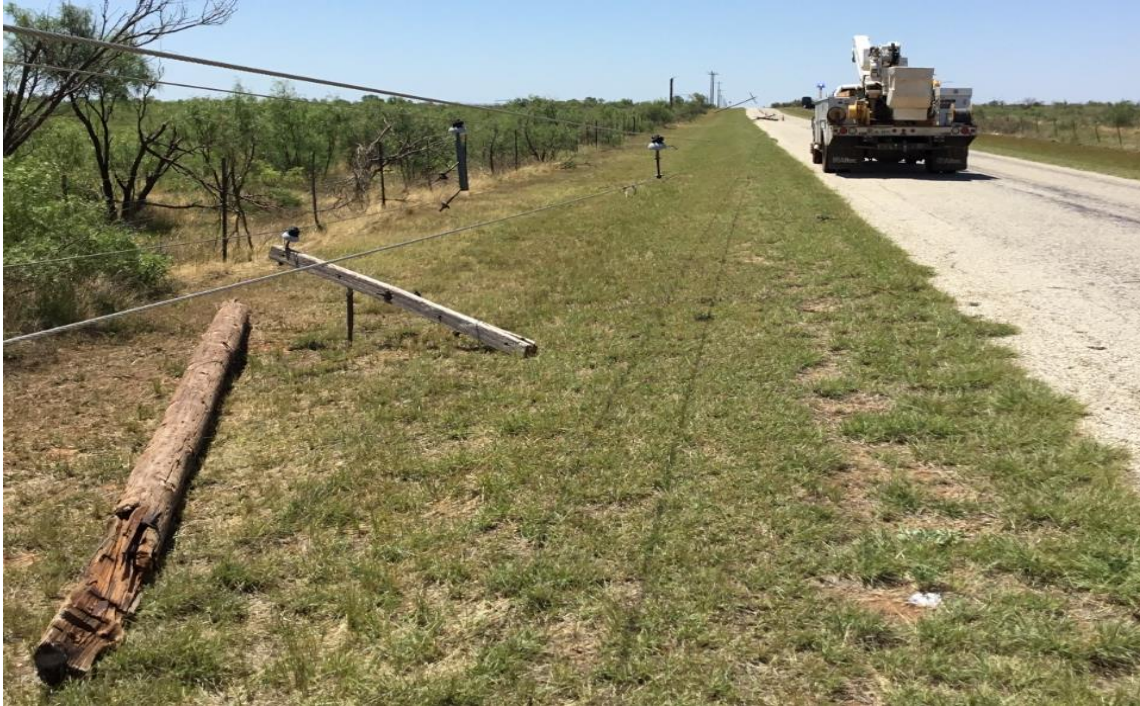
Figure 6: Downed powerline poles along Willow Valley Road. All of the poles were snapped in half.
