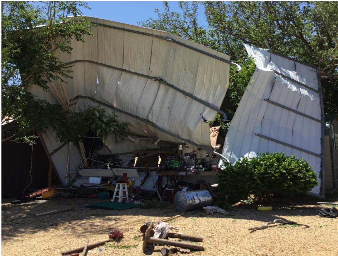
Figure 5: A large metal shed also located on the southeast side of Gail, TX, was overturned and ripped in half.
