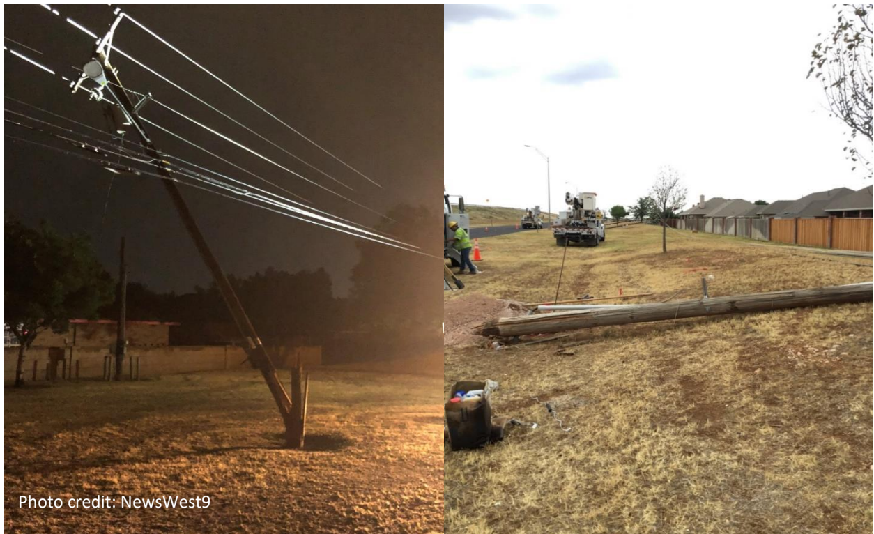
Figure 3. Wood powerline poles snapped at their base and leaning over along the westbound frontage road of Andrews Highway.
