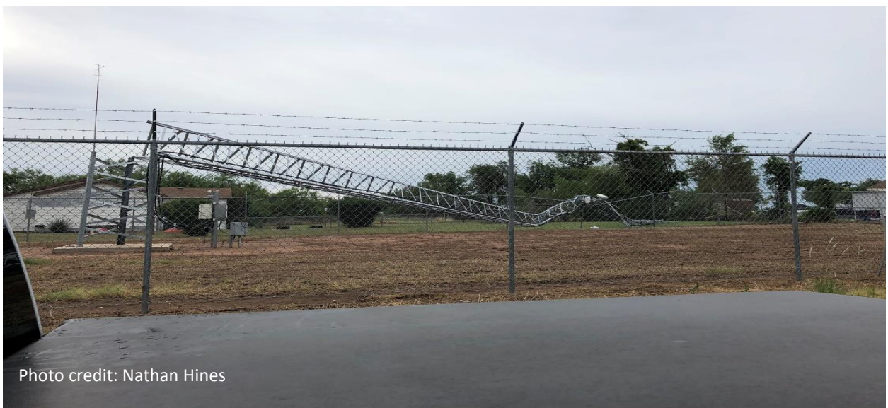
Figure 5. 100 ft tall radio tower in Snyder, TX broken near its base due to strong straight-line winds.
