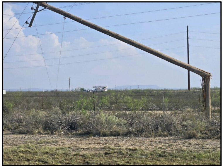
Photos of hail damage to a home and a snapped power pole due to straight-line winds. Photos are courtesy of Kendra Reed and Pecos County EM.
