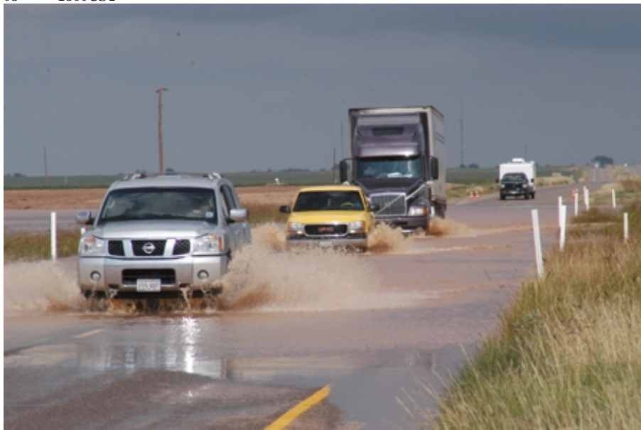
A flooded playa lake inundated a section of U.S. Highway 87 north of Lamesa for more than a week during early October. Traffic was detoured at times to smaller state routes. The driving surface was severely damaged by the time flood waters receded on October 8th. Photo Courtesy: Russel Skiles - The Lamesa News - Reporter.
