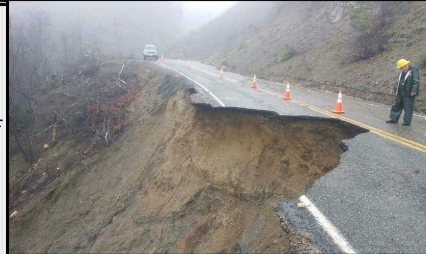
*At left: Gaping hole opens up beneath Highway 42s east of Bandon. (Photo: ODOT)*
