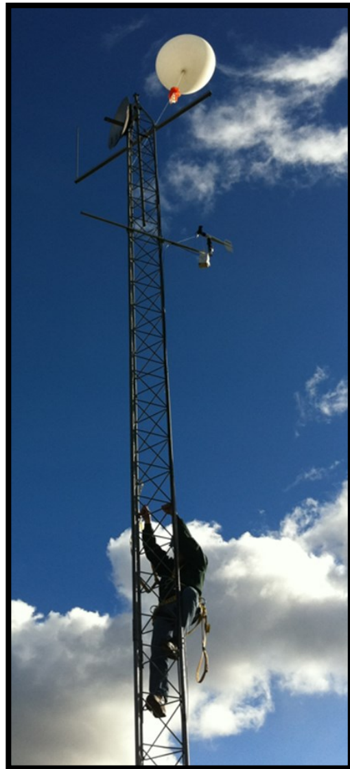
NWS Electronics Technician climbs the observation equipment tower to free a stuck balloon from a botched balloon launch.
