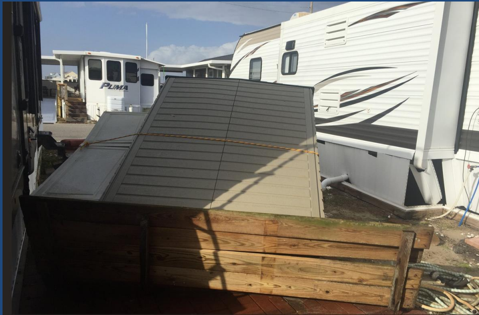
Thunderstorm Wind Damage in Emerald Isle, December 20, 2018.
