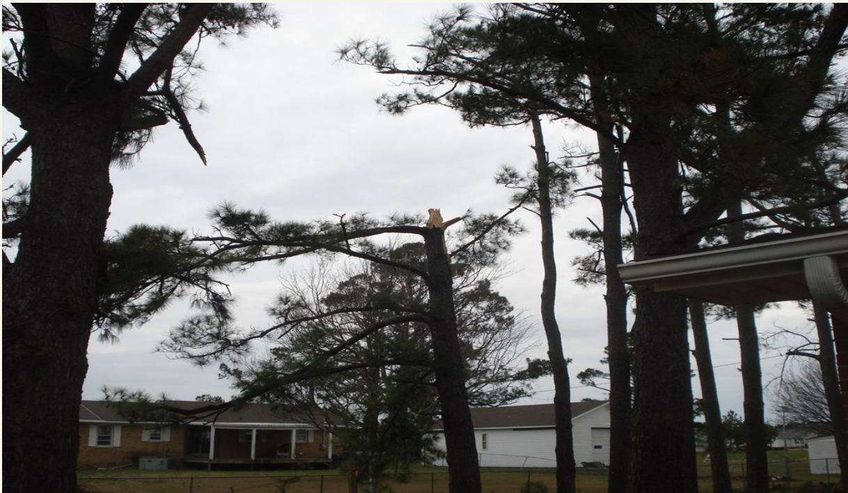
Damage at Merrell home (Merrell family photos).
