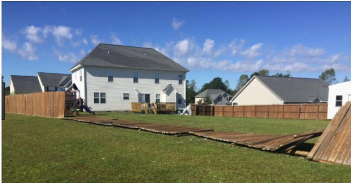
Minor Wind Damage in Richlands, NC, October 24, 2017. Photo from WCTI TV.
