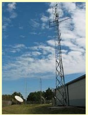
GAP Voyager, CL33 rotatable beam & VHF tower
