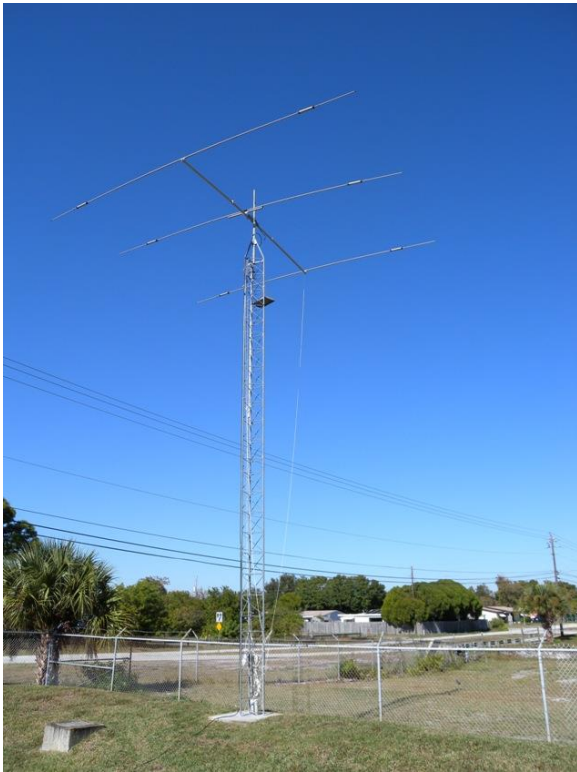
CL-33 rotatable beam
