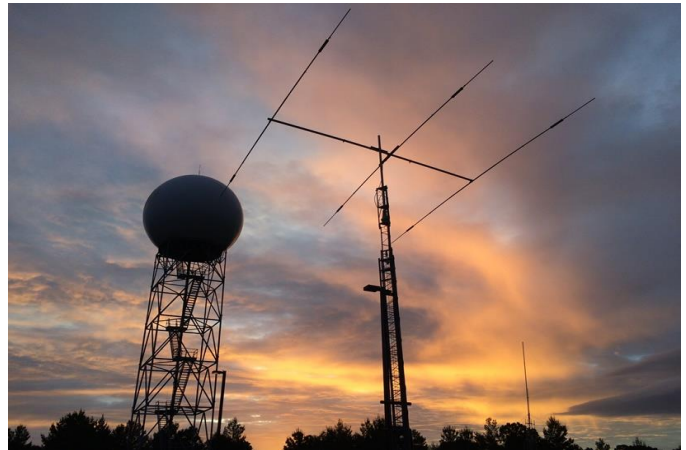
KMLB WSR-88D Radar and CL-33 Rotatable Beam
