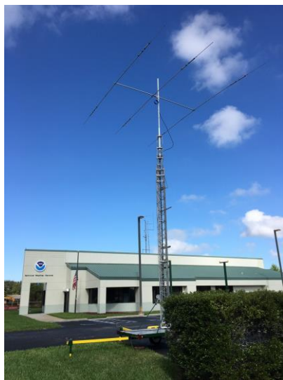
MCARA tower and A-3S Rotatable Beam
