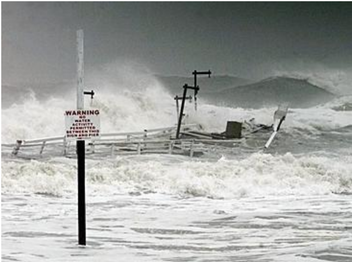
Daytona Beach Main Street Pier collapsing
