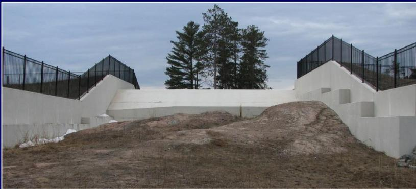
At Tourist Park, a new dike and spillway have been constructed where the new river channel was carved out during the flood.
