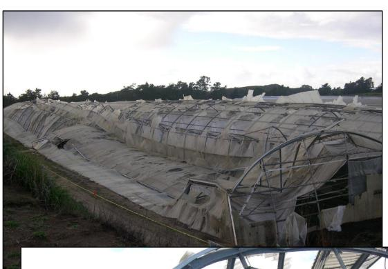
Significant damage to greenhouse structure on commercial farm at point B on map. Images from NWS Damage Survey.
