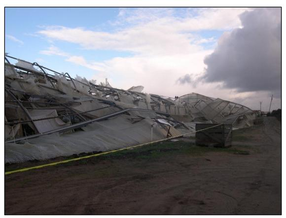
Damage to greenhouse structure at commercial farm showing collapsed metal structure and fiberglass/plastic sheeting damage.
