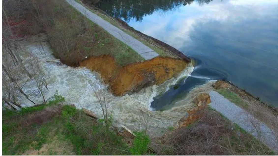
Dam failure in Putnam County, Tennessee in April 2020
