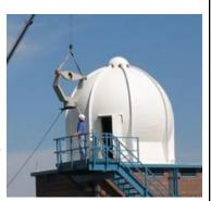
Out with the old and in with the new, here is the new RRS antenna being installed within the domed upper air building at the NWS Spokane office.
