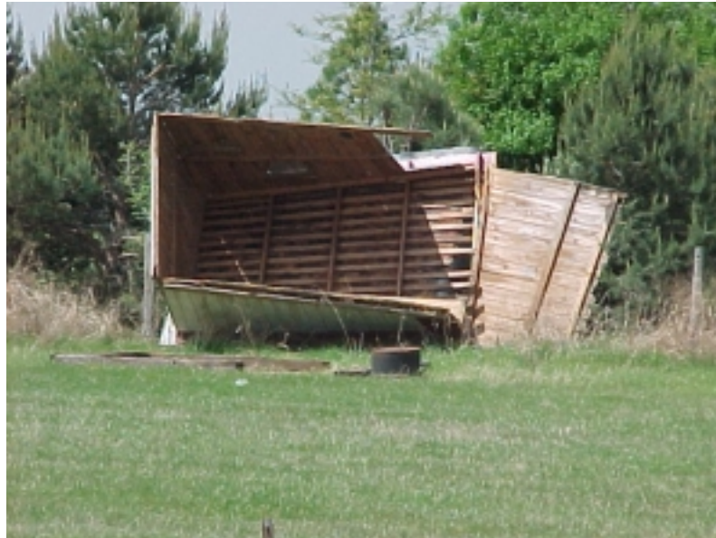
Wooden outbuilding rolled intact onto its west side 1.5 miles southeast of Morrison.
