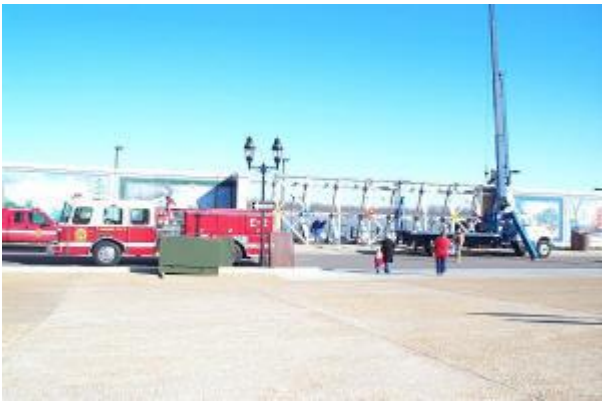
Firefighters and other city workers install a floodgate in downtown Paducah, KY on January 14. This was the first time since the 1997 flood that floodgates were installed in Paducah.
