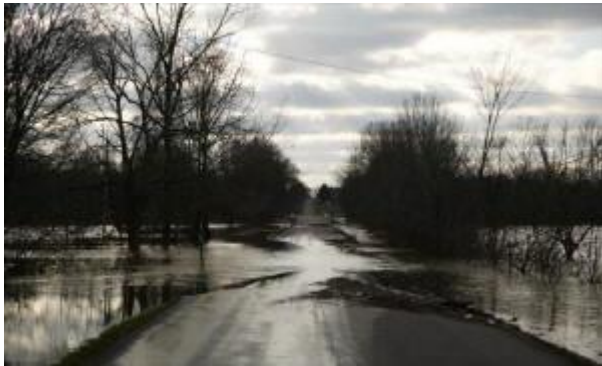
Water covers a road in Livingston County, KY. Photo from Beau Dodson.
