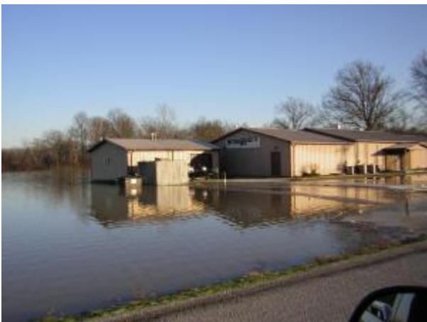
Water begins to surround a restaurant in Harrisburg, IL (Saline County). Photo courtesy of Tracy Felty.
