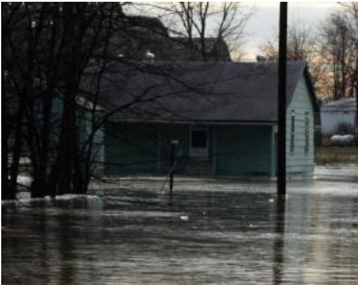
Photo of a flooded area on Pearl Street in Metropolis, IL. Photo courtesy of Beau Dodson.
