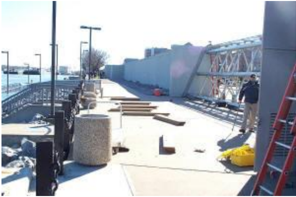
Another photo taken on Friday, Jan. 14 of the floodgate installation in downtown Paducah.
