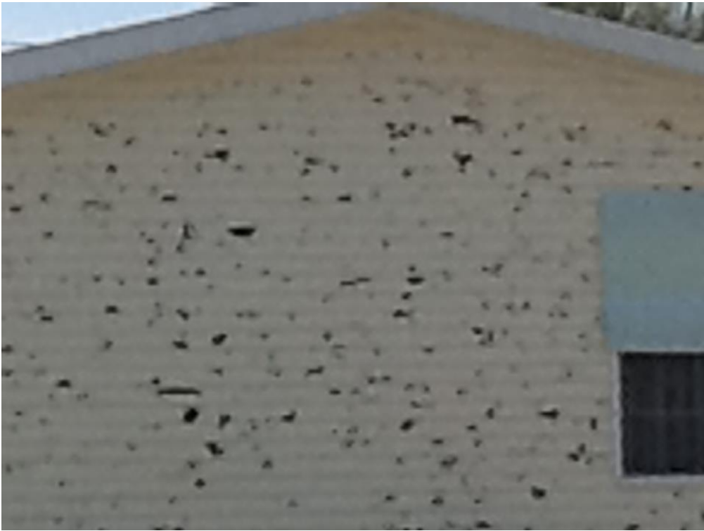
Hail damaged home in Oakland City
