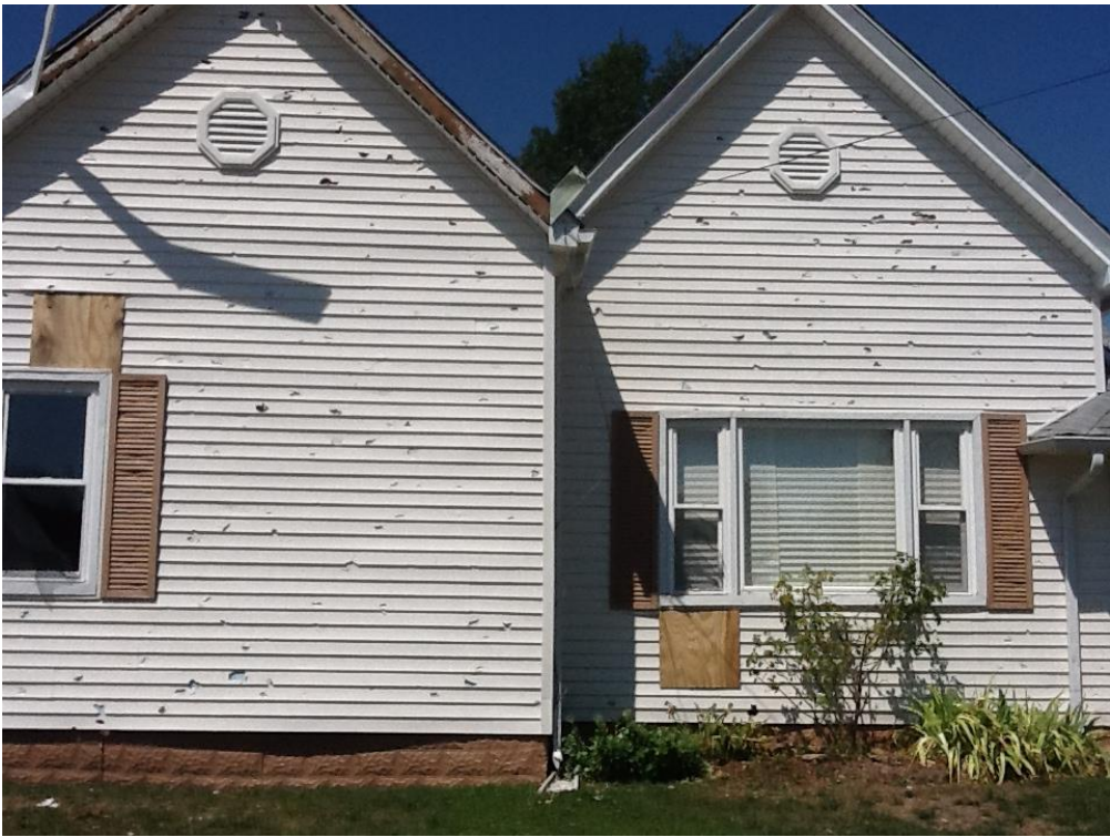
Home damage in Oakland City
