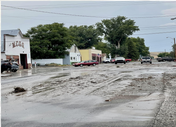
Left over mud after heavy rain flooded Lone, OR
