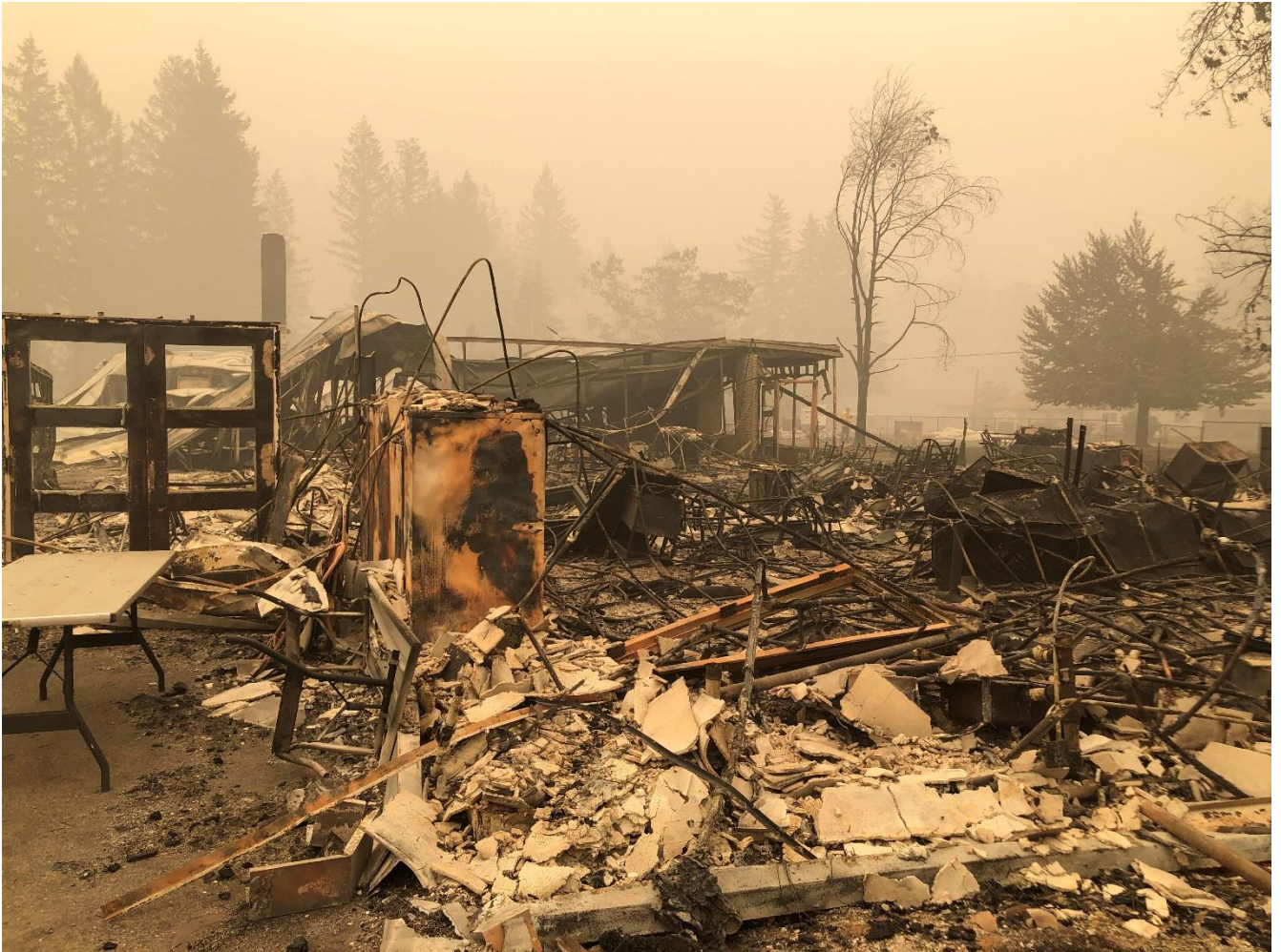
Gates Elementary School – FBAN and IMET work area in the back end
